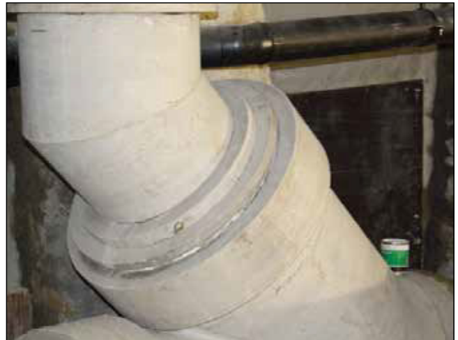
Figure 32 - Example of SuperTite Reducers used to change pipe diameter
